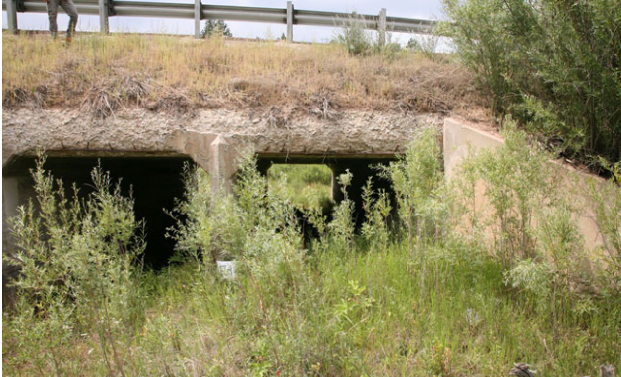
Picture 2 – Bridge I-15-AO Downstream
