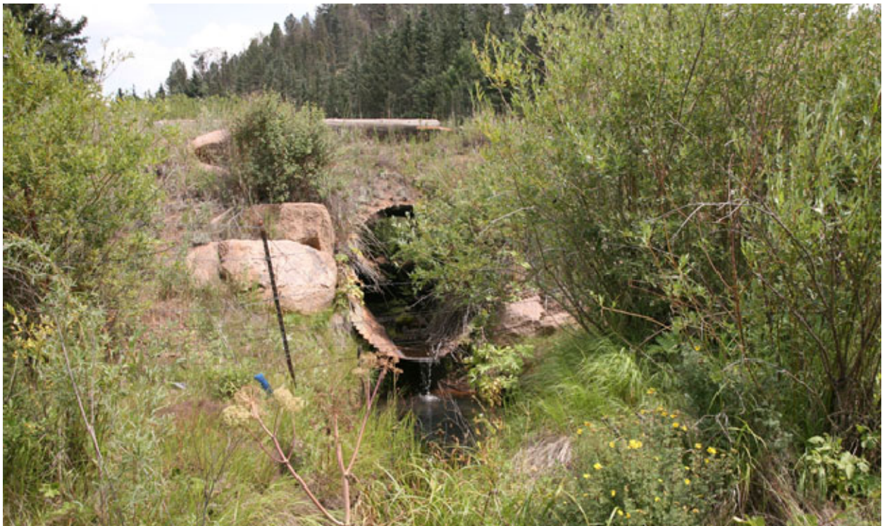
Picture 3 – Pipe Upstream
