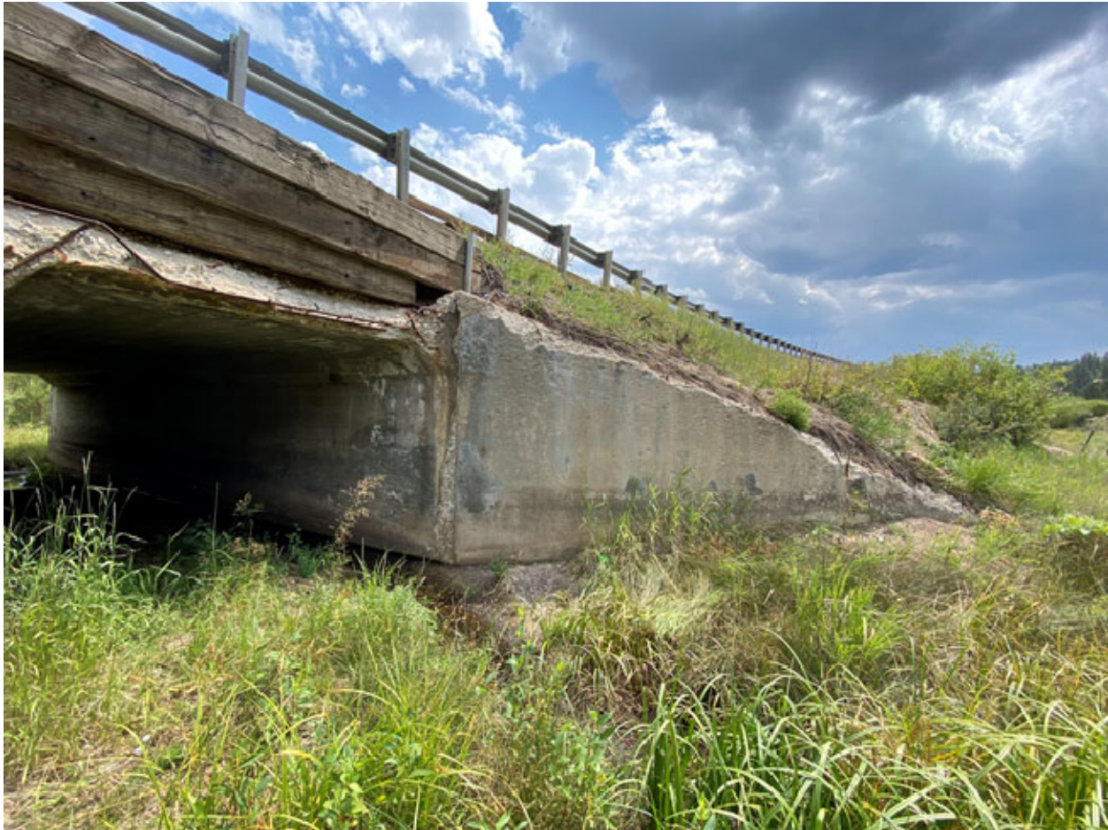
Picture 1 – Bridge I-15-AO Upstream
